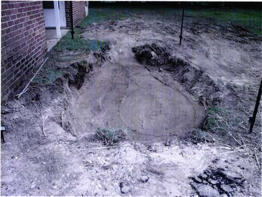
# 7 Bay Circle- During compaction testing
