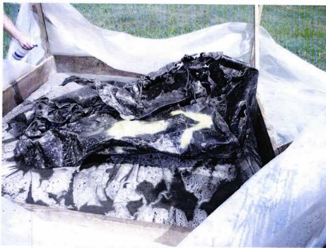
# 7 Bay Circle- Tank 7-1 being cut and deconed.
